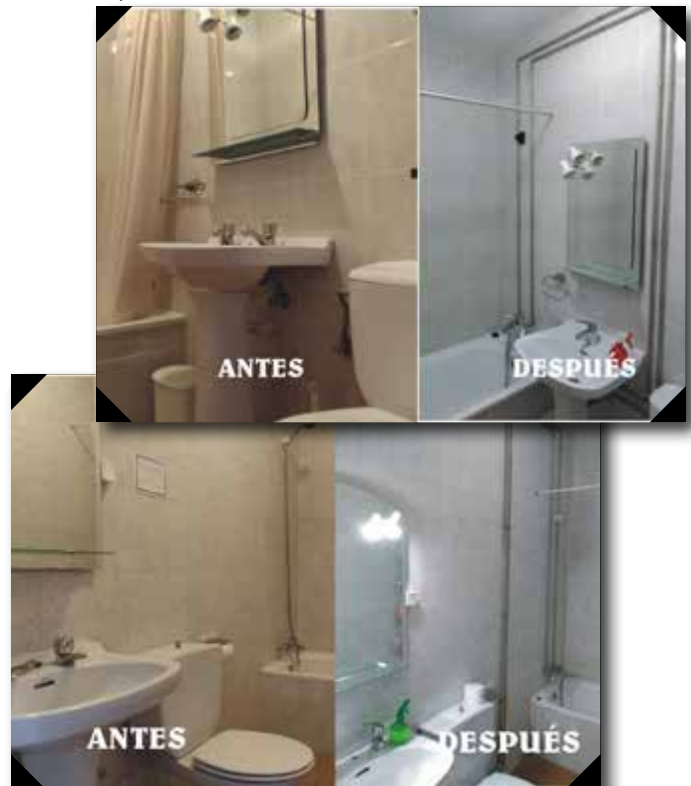
Before and after photos showing replacement of the hot and cold water system in 2020 at the Albergue de la Santa Cruz, Sahagún.
